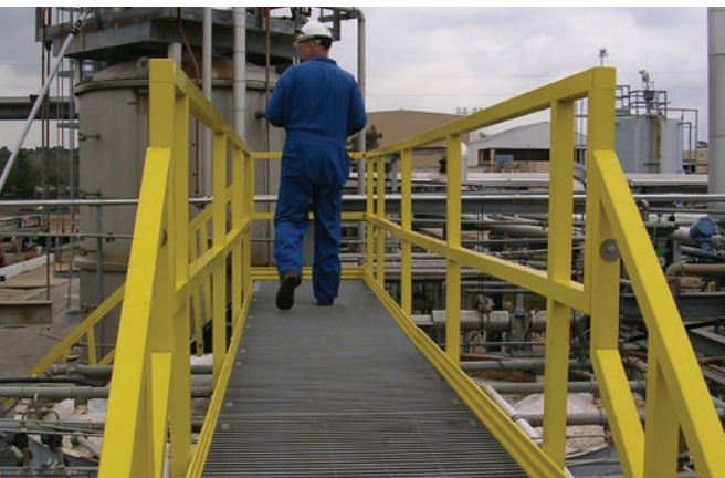
SAFRAIL™ and DURAGRID® pultruded grating were fabricated to make access platforms over wastewater recycling tanks. The previous steel structure corroded, and was unsafe.
