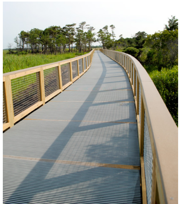
Almost 5,000 panels of I-4000 1" were used to create a nearly half-mile walking and biking path at Cape Henlopen State Park near Lowes, Delaware.
