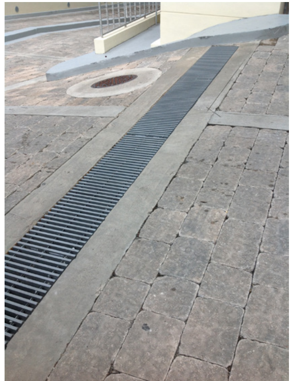
HD-5000 1-1/2" was used at a high-end condominium complex in Miami Beach, Florida to cover drainage channels at parking garage entryways.
