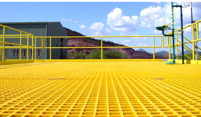
Corrosion resistant DURAGRATE® installed around the solvent extraction electrowinning (SXEW) process of a copper refinery in Piedras Verdes, Mexico.
